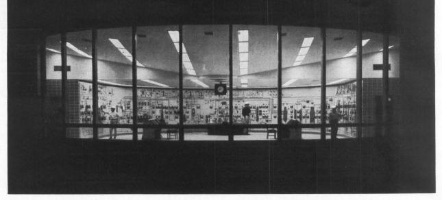
**Compactness of DDC** will replace such massive nerve centers as this Central Control House at Sohio's Toledo Refinery. Instrumented 96-foot curved panel controls processing loops and catalytic cracking and steam generation
