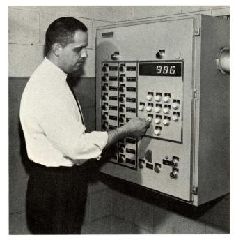
Remote input/output panels provide on-the-spot operator-process communication.
