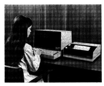
The Hazeltine 2000 is the most popular display terminal of the six models offered by the company. Included with the terminal shown above is the optional 30 cps thermal printer. The Hazeltine 2000 is marketed as a direct replacement for Teletype Model 33 and 35 units.
