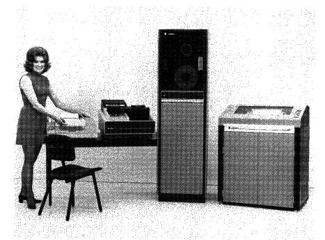
A typical Unitech UT-1 configuration includes (from left) an operator console (Teletype Model 33 ASR), card reader, optional magnetic tape drive, and line printer. The Data General minicomputer is housed in the central cabinet along with the tape drive.
