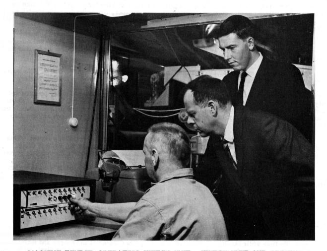
MACHINE TENDER OPERATING SWITCH UNIT. SWITCH UNIT AND PRINTER PLACED IN THE MACHINE TENDER'S BOOTH AND ARE USED TO COM-MUNICATE WITH THE COMPUTER. The purpose of the control system is to attain the above objectives by automatic control action and by assisting the machine tender in the execution of manual operations when required.
