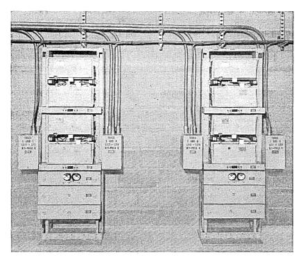
Fig. 17 — Typical auxiliary repeater in concrete block nut.
